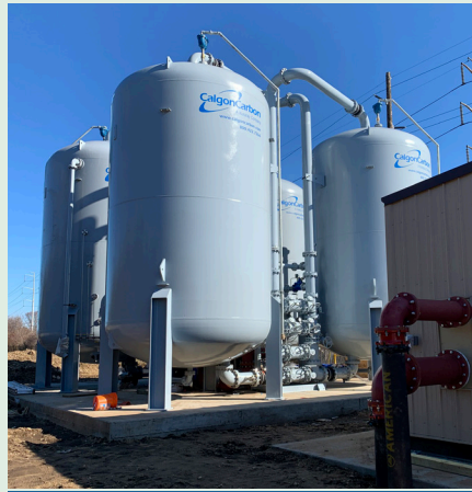
Recently installed GAC vessels at one of the District's plant sites
