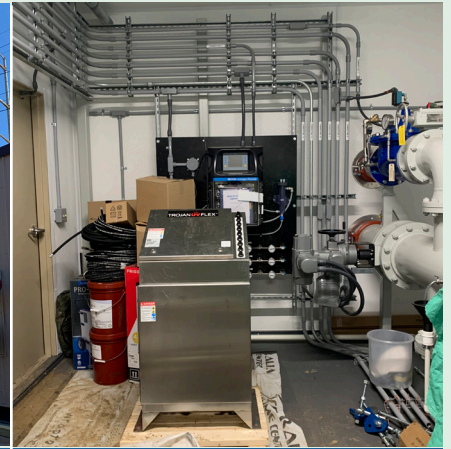
AOP unit that will be removing 1,4-dioxane from our water
