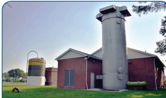
Hicksville Water District Plant 6 was awarded the 2014 Project of the Year (Medium System) by the New York American Water Works Association.
